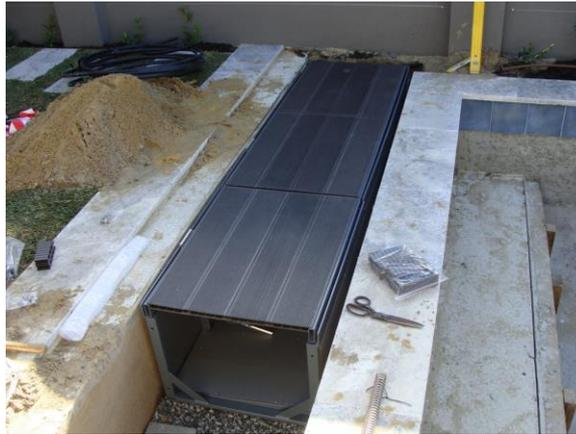
6. Starting from one side, line up the Module frame joints with the next module (refer to packing label from step 1 for sequence). Check that the top of the Module decking is level with the finished level of the paving. Unclip electrical joiners and leave hanging
