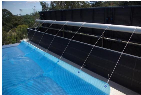
32. Ensure the cover is recovered correctly, roll and unroll cover a number of times to make sure your Showcase is in the correct position. On the right and left modules only, drill through 4 x anchoring points with supplied masonry drill bit, insert and secure 4 x masonry anchors
